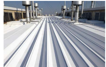
Thermal insulation paint on the roof of the Saitama Plant
